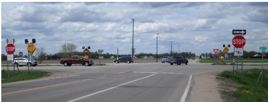
Looking north at Highway 23 and CR 7.
